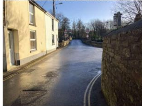
Figure 8.5 North Street / Grenville Road – Lostwithiel Bridge
