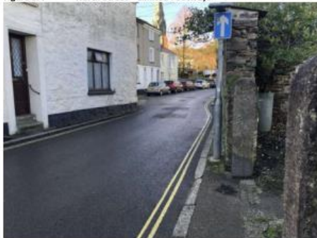
Figure 5.4 North Street – Limited Footways
