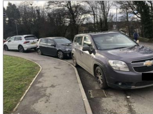
Summers Street – Two vehicles parked blocking access to utilities where 'no parking signs are displayed.
