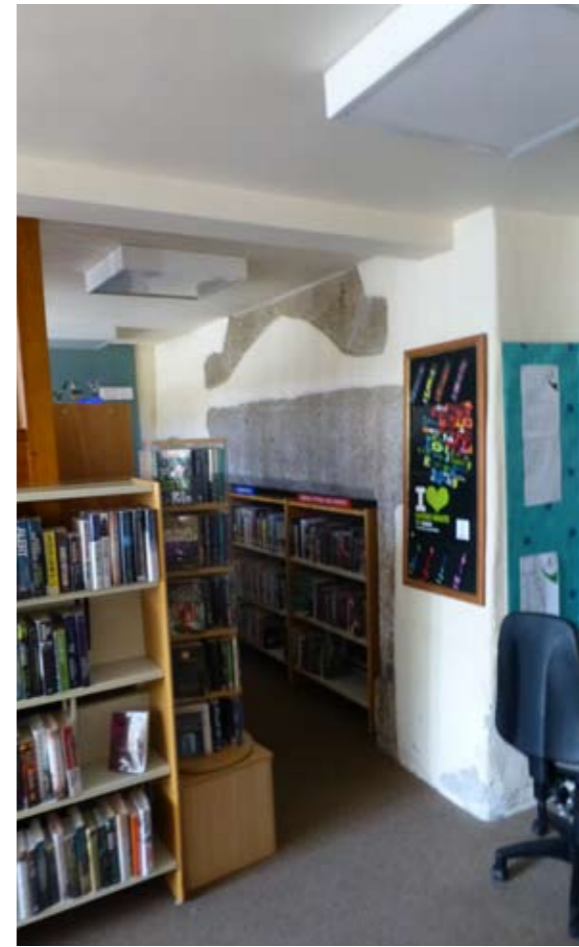
Taprell House internal details
