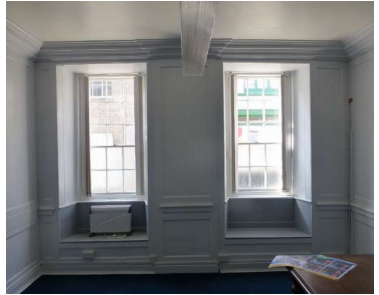
Internal view of ground floor room
