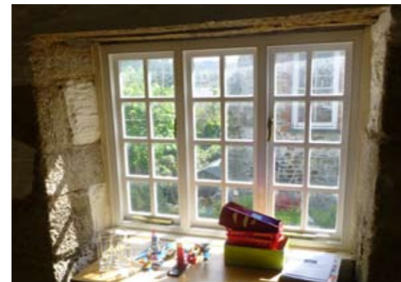
Existing window features in Taprell House
